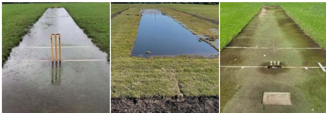
Figure 25. The relative levels of the wicket and surrounds at these sites are incorrect, resulting in water ponding on the wicket and causing match cancellations. To allow wickets to drain, the surrounds 2m from the wicket should be 40mm lower than the pitch.
