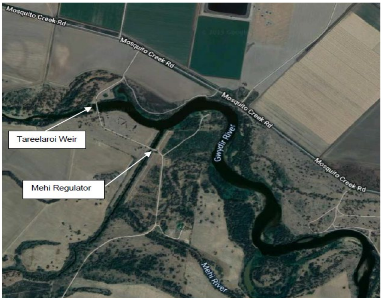
Figure 2. Location of Tareelaroi Weir and Mehi regulator
