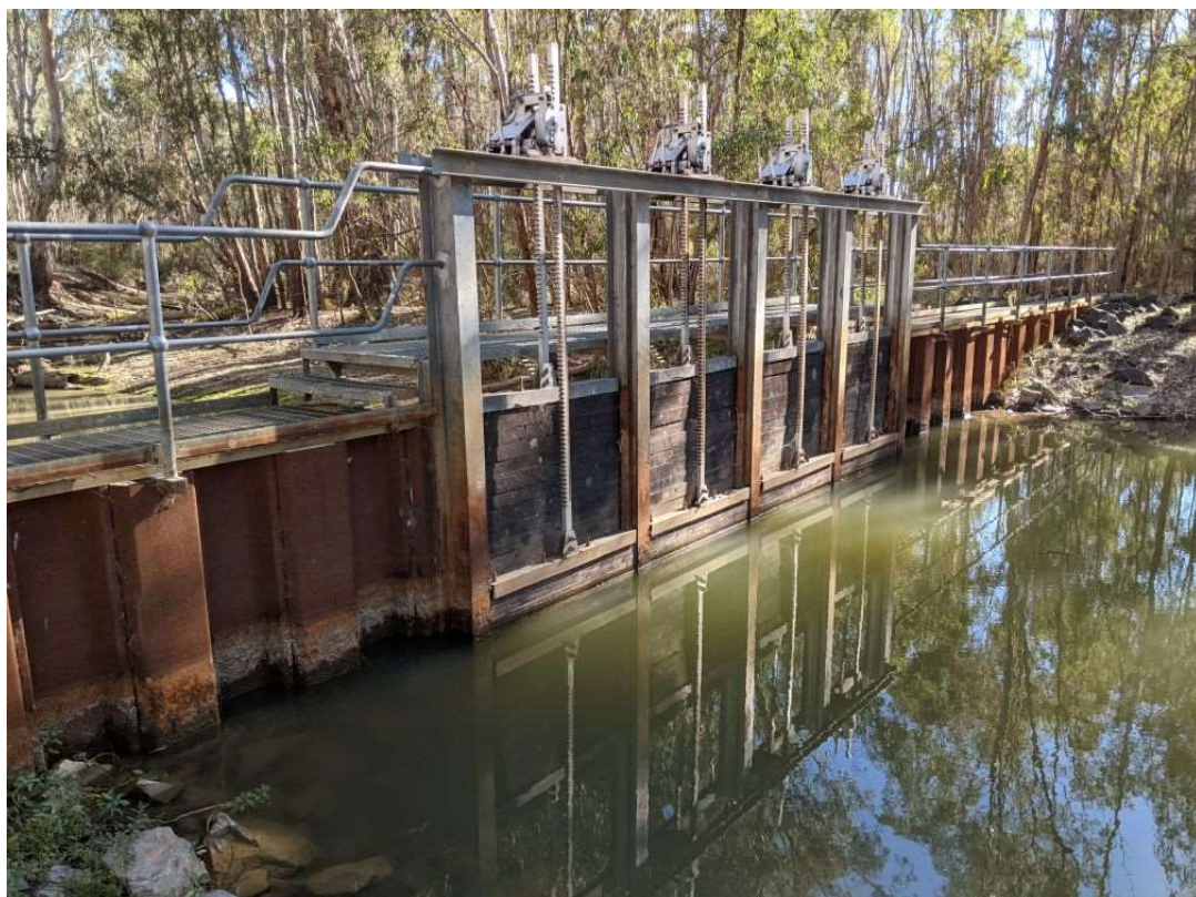
Photo 2-13 Existing Little Edward River offtake regulator – upstream
