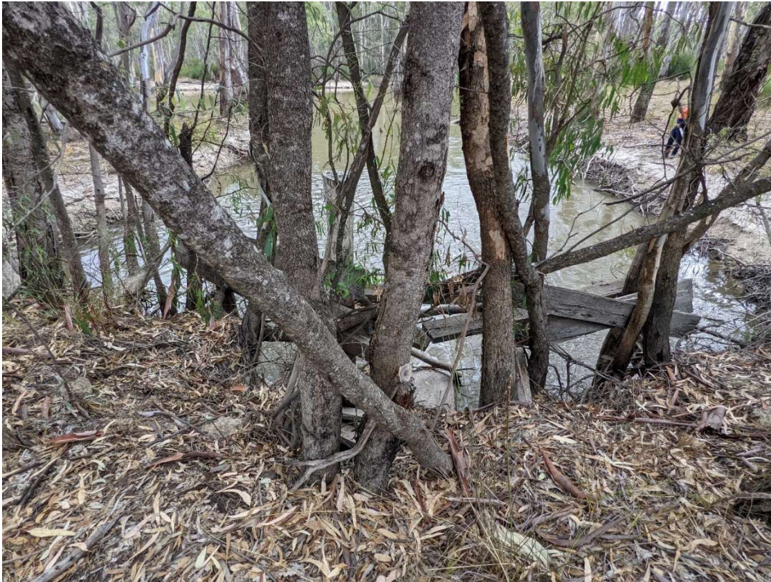
Photo 2-19 Existing Pigsty culvert facing downstream along Pigsty Creek towards where it joins the Edward River
