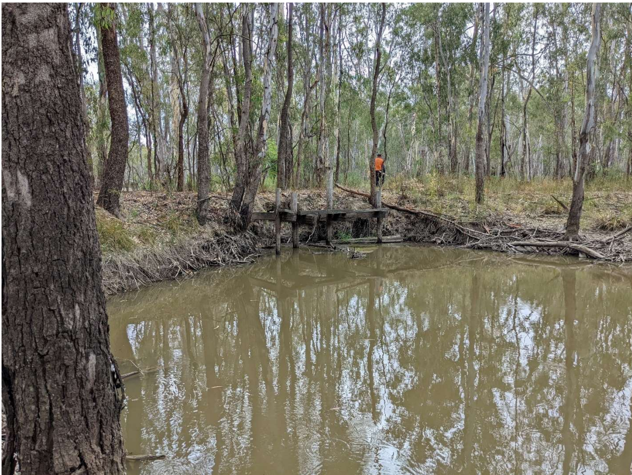
Photo 2-15 Existing Pigsty culvert in higher flow – upstream
