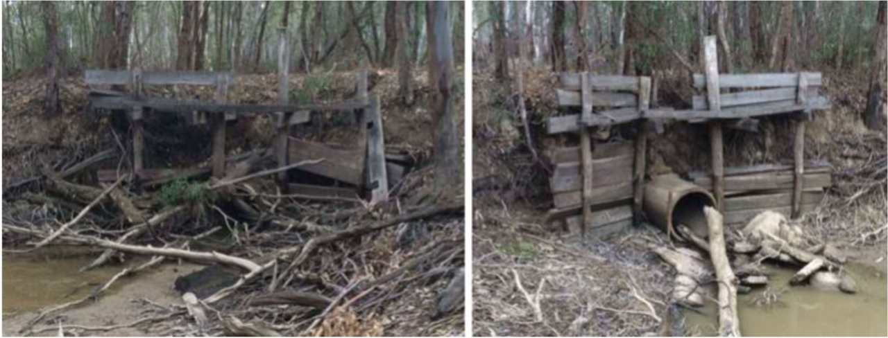
Photo 2-14 Existing Pigsty culvert in low flow – upstream (left photo) and downstream (right photo)
