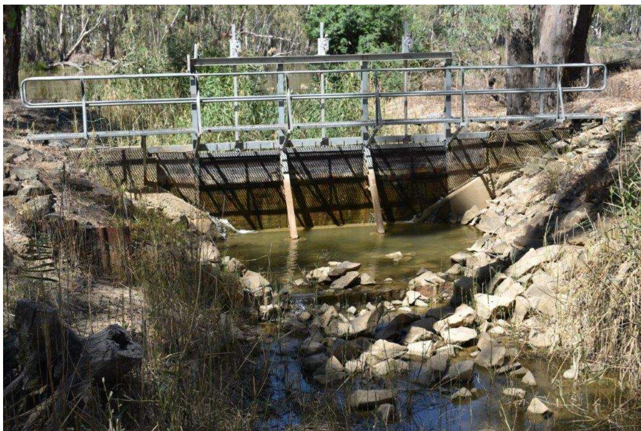
Photo 2-6 Existing Nestrons regulator, downstream
