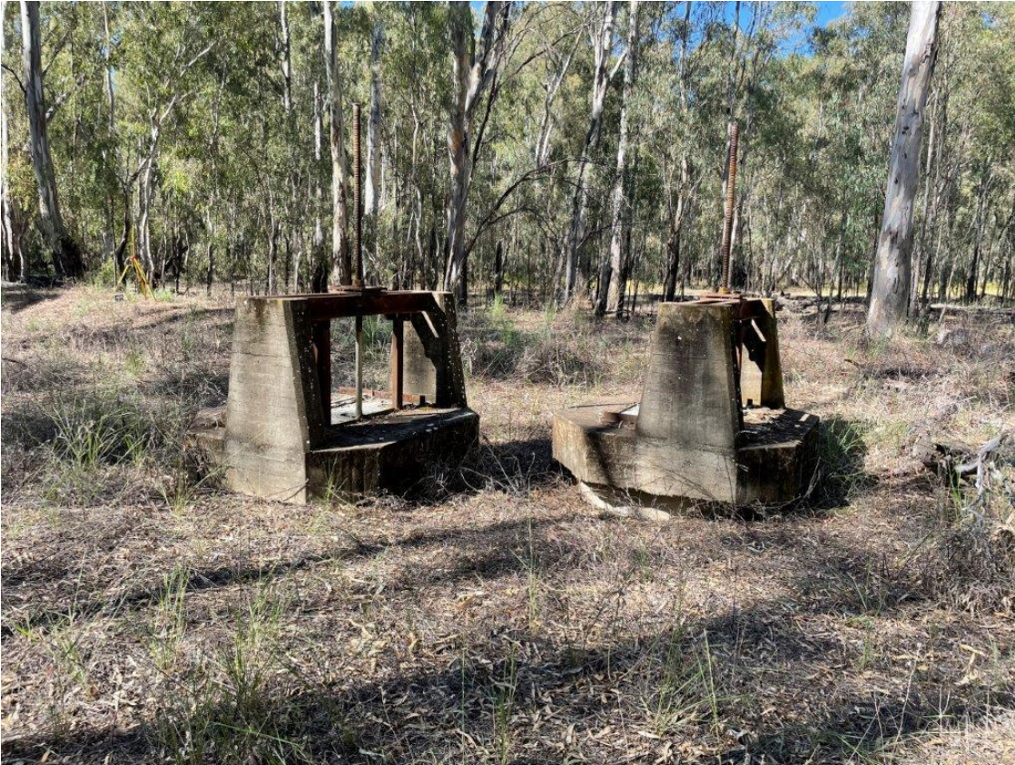
Photo 2-4 The penstock gates of the existing inlet regulator
