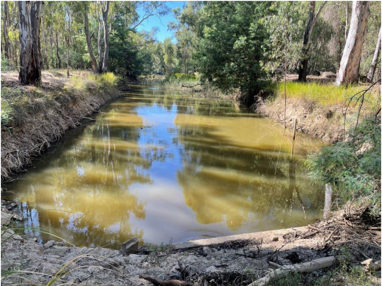
Photo 2-1 Bullatale inlet channel, looking upstream from the inlet regulator towards the Murray River. The top of the inlet regulator is just visible above the waterline at the bottom of the photograph
