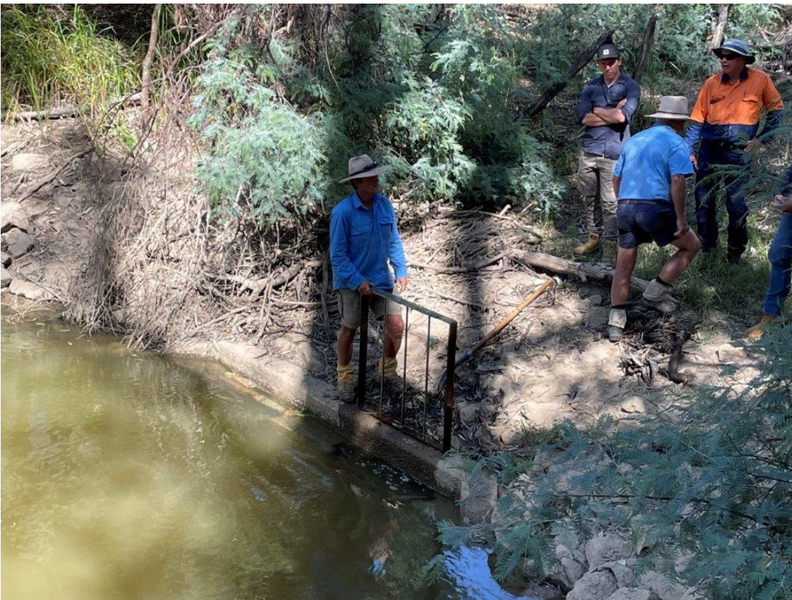
Photo 2-5 The penstock gate at the upstream end of the existing inlet regulator
