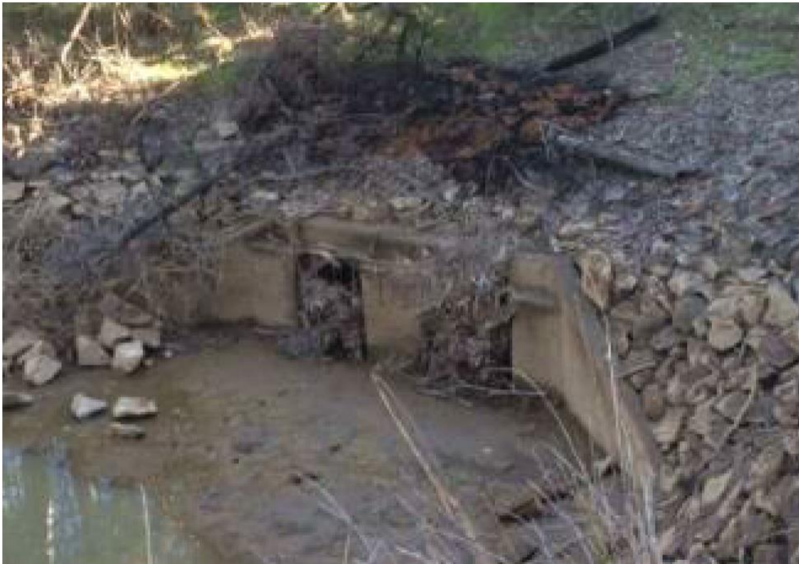
Photo 2-6 The upstream end of the existing inlet regulator, shown when there is no flow in the inlet channel
