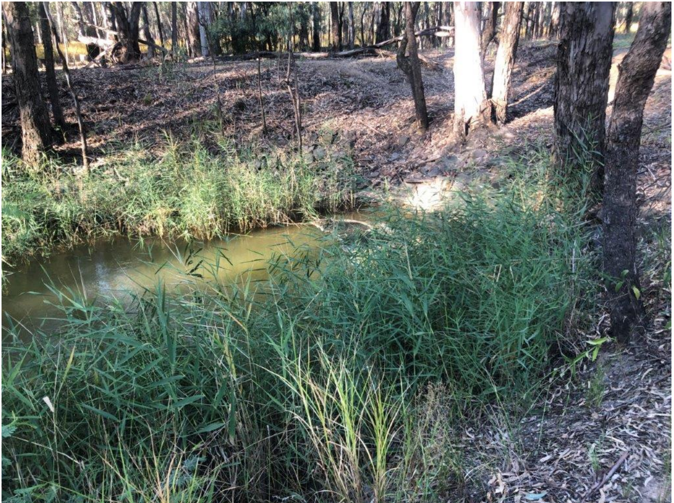
Photo 3-1 The downstream end of the existing inlet regulator, where the buried twin pipelines discharge flow into Bullatale supply channel
