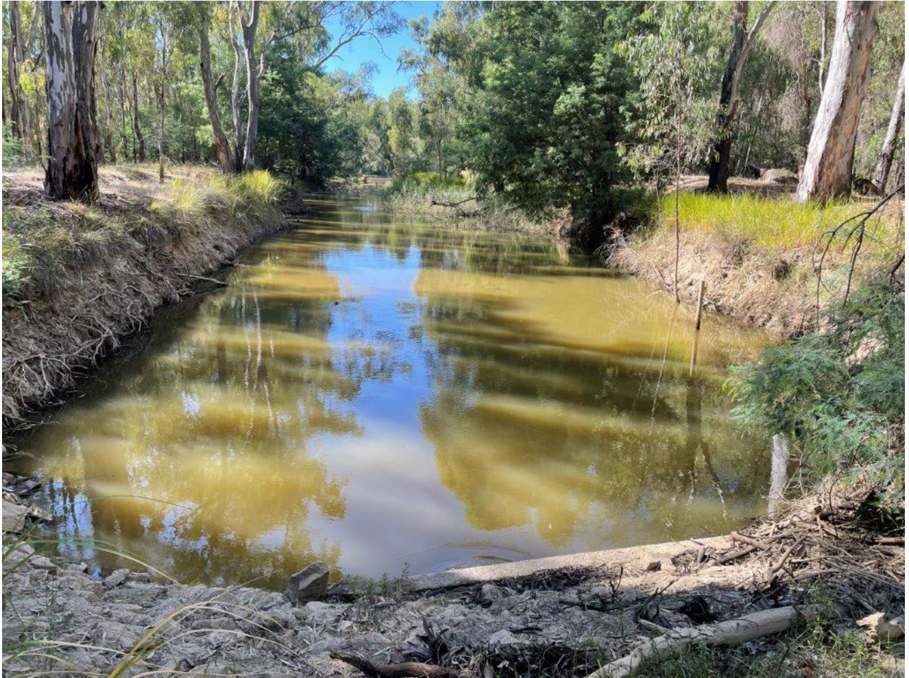
Figure 2-1 Bullatale inlet channel, looking upstream from the existing inlet regulator towards the Murray River. The top of the inlet regulator is just visible above the waterline at the bottom of the photograph.
