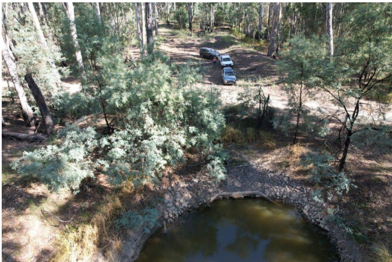
Figure 2-2 Bullatale inlet channel, looking downstream across the existing inlet regulator and constructed embankment
