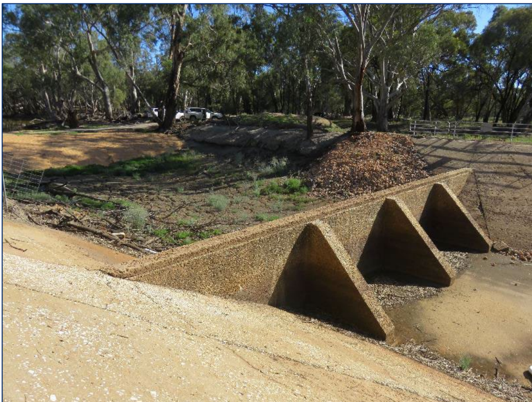
Figure 2-2 Existing Carrs weir No.2 structure (with upstream coffer dam)
