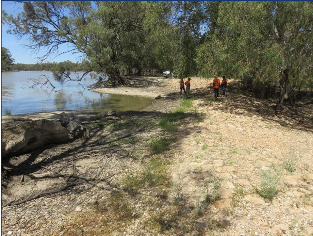
Figure 2-6 Existing block bank at Mike's Runner (Site B) with River Murray on left
