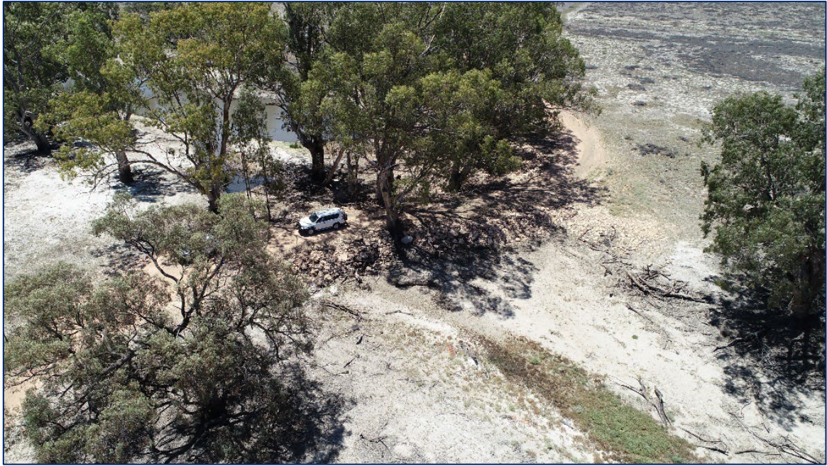
Figure 3-2 Site 9 (Bunberoo Creek) – existing causeway site and clearing for new bridge
