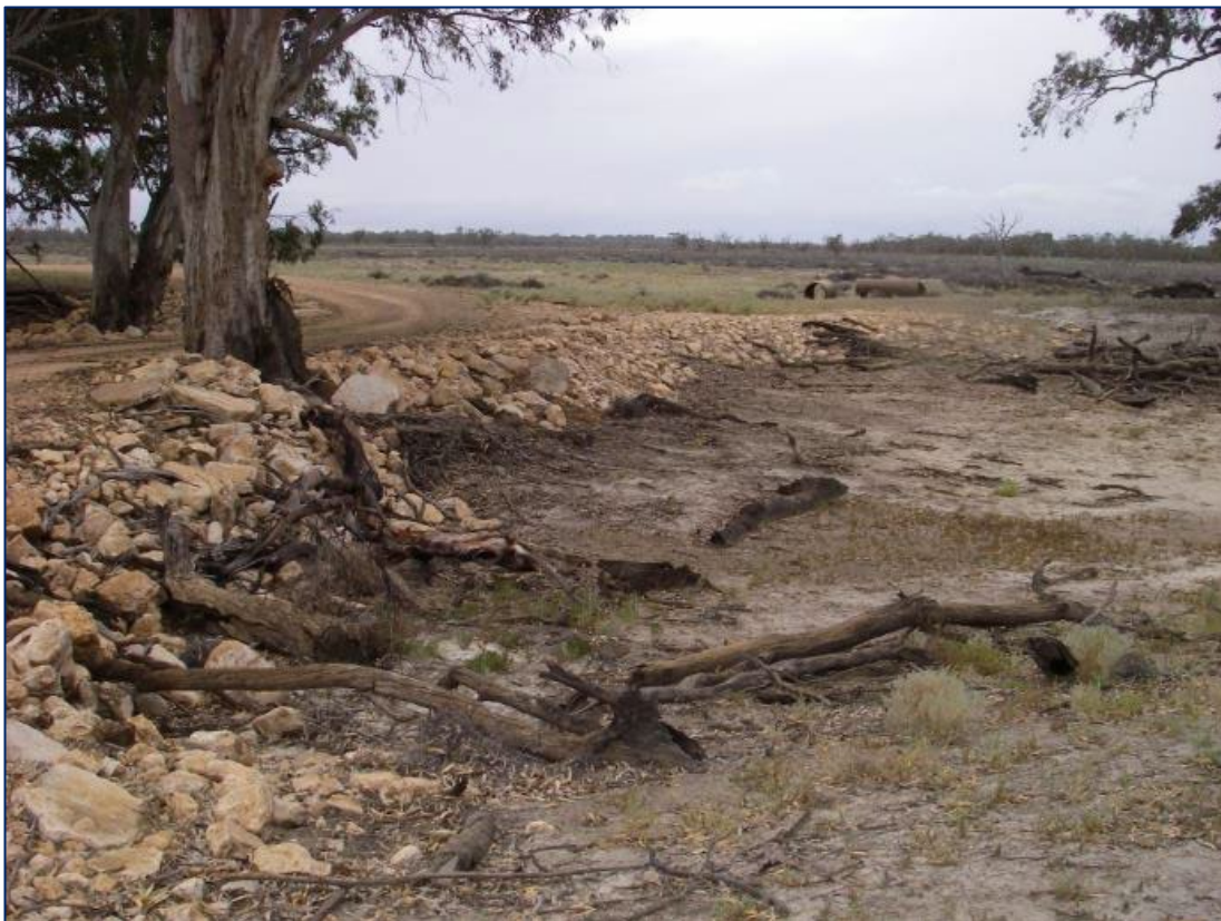
Figure 2-5 Existing Bunberoo Creek crossing at Site 9 (eastern side of causeway looking north)
