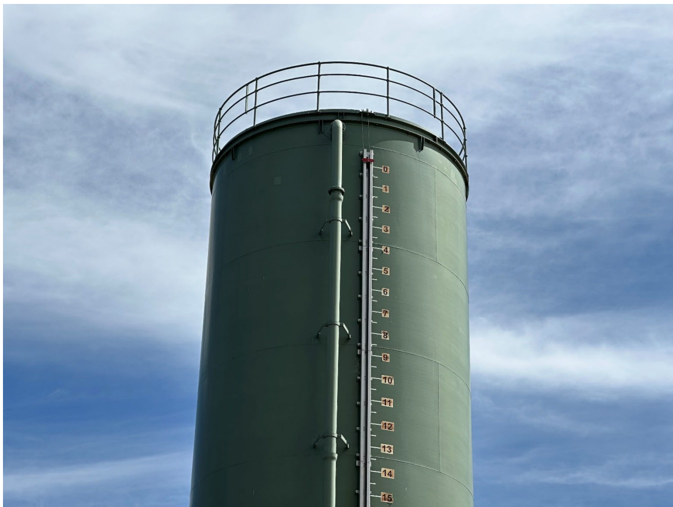
Image 2 A water tower in regional NSW.
