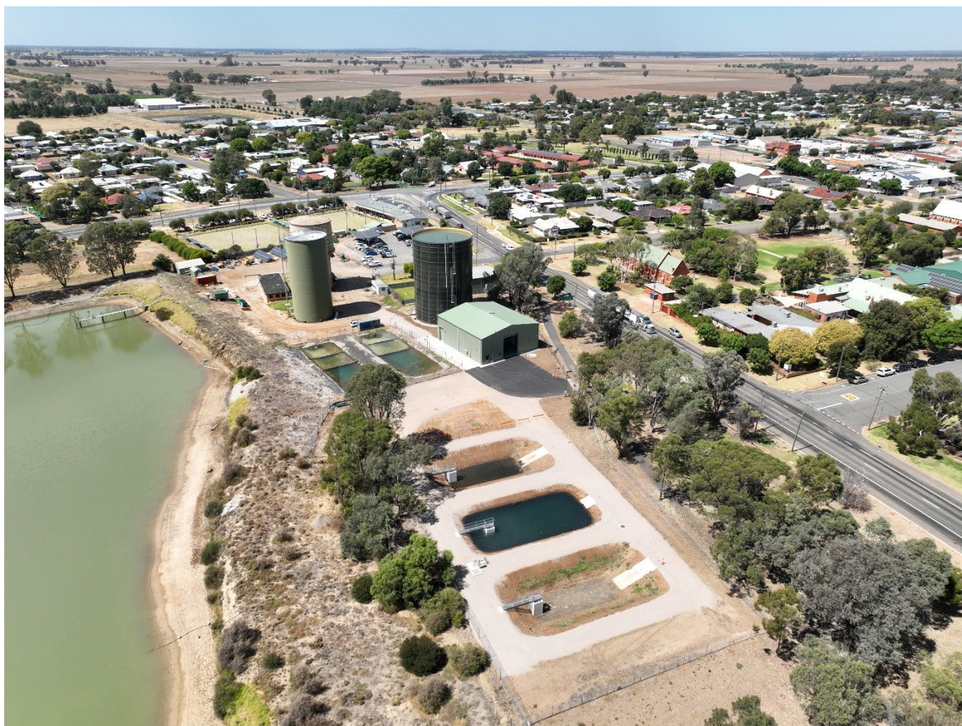
Image 1 Aerial view of a water treatment plant in Finley, NSW.
