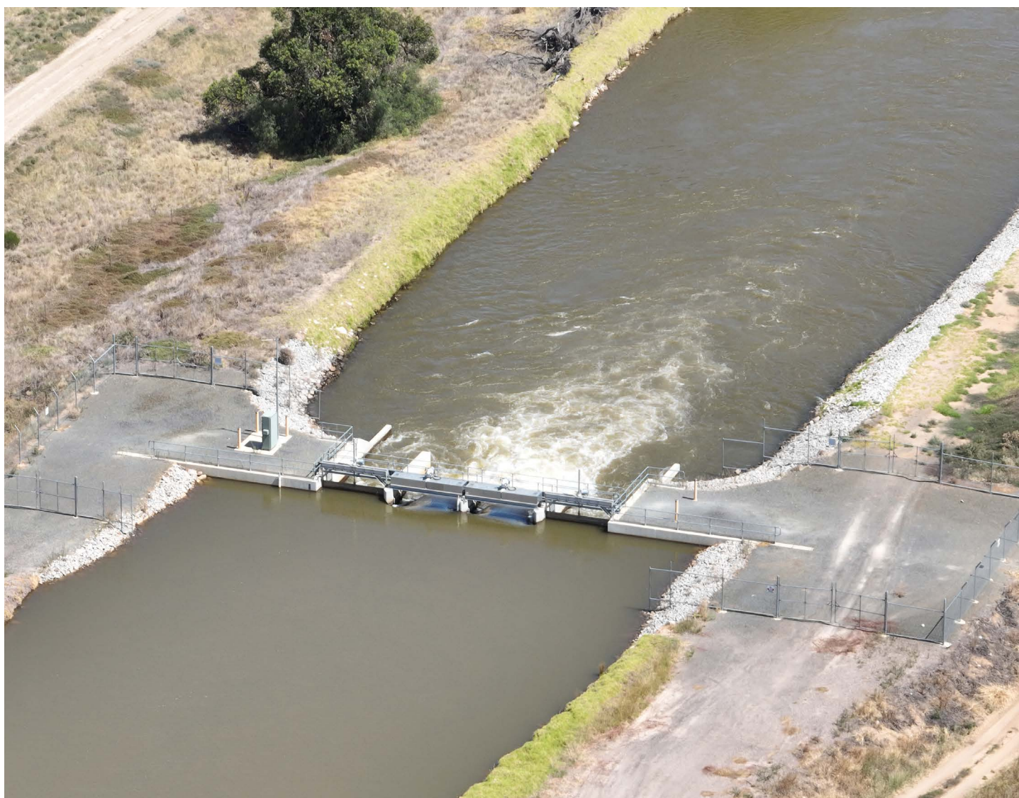
Image: Mulwala canal at Finley. Photo: Vince Bucello.
