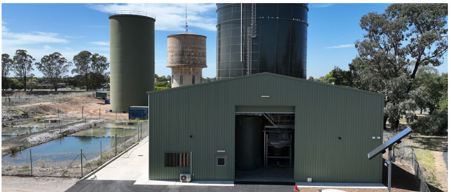
Image: Finley water treatment plant. Photo: Vince Bucello.
