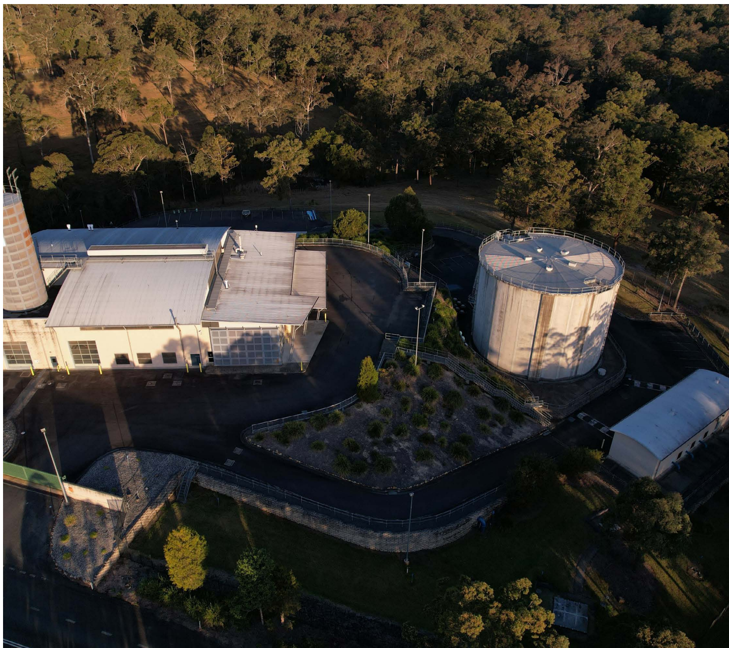
Image: A bird's eye view of a water treatment plant in regional NSW.
