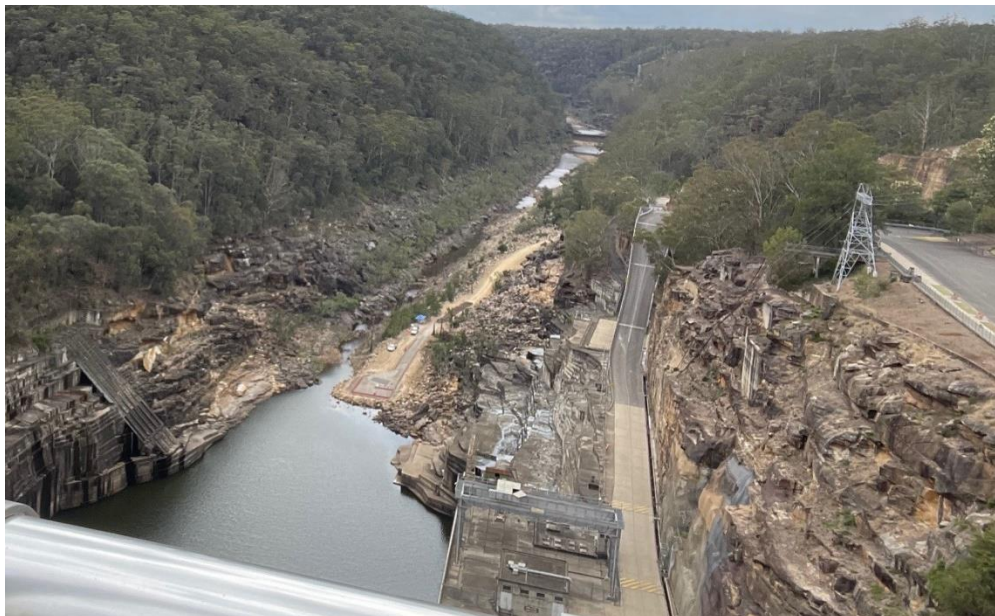
Figure 3: View from atop of Warragamba Dam.
