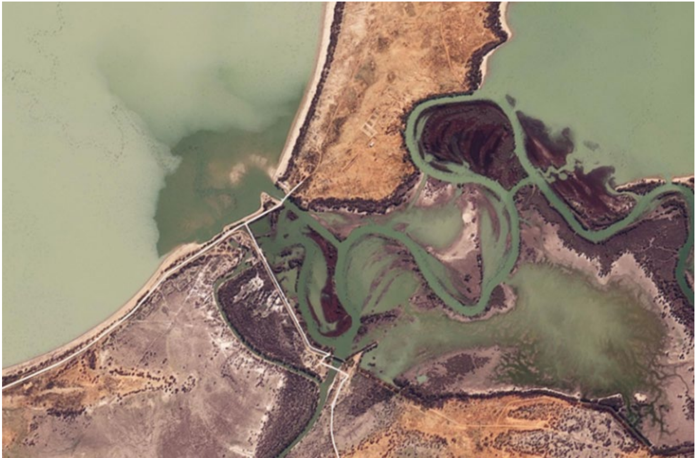
Figure 1. Satellite image of the Pamamaroo inlet regulator highlighting the location of the hook shaped sediment bank and the water from Lake Wetherell not dispersing into the lake – 5 August 2026
