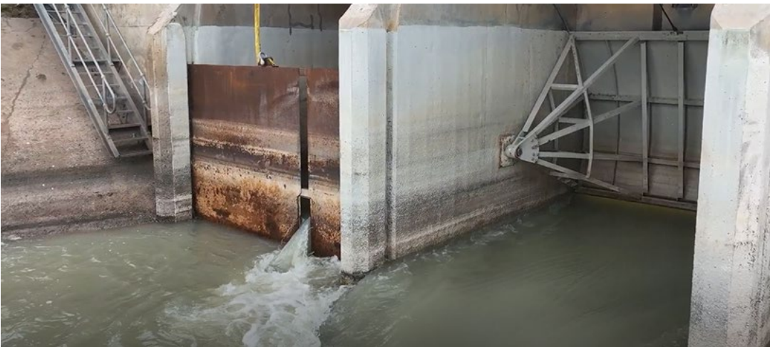
Figure 2. Fish baffles being installed at Pamamaroo Inlet Regulator – August 2026
