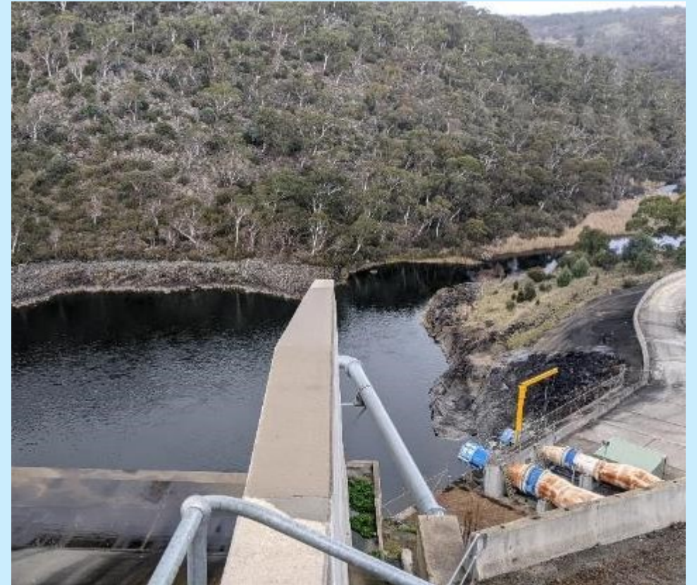
Image: Snowy River from Jindabyne dam showing cone valves for environmental releases
