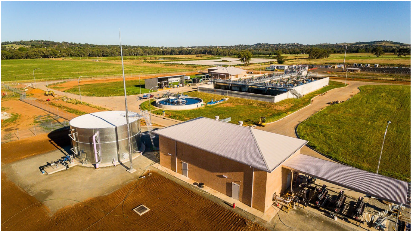
Figure 6. An aerial photo of the Parkes Shire Council's Recycled Water Scheme that supplies water for municipal irrigation around Parkes (Courtesy of Parkes Shire Council)
