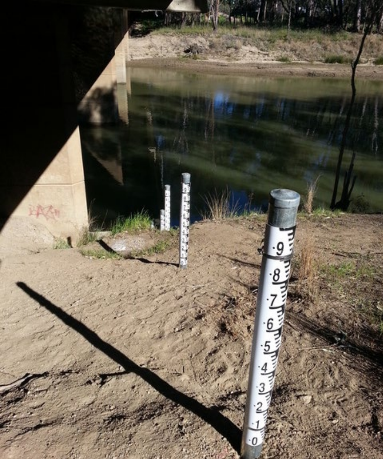
Darlington Point gauge location
