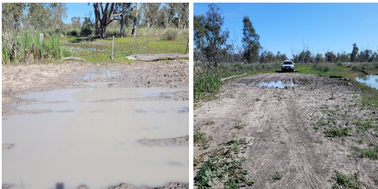
Figure 2-2 Existing low-level crossing on Bronzewing Drive
