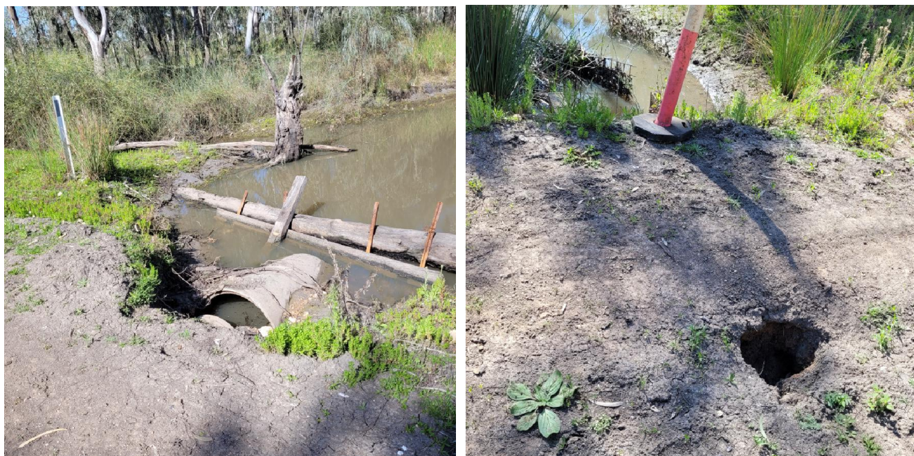
Figure 2-3 Existing pipe culvert on Bronzewing Drive
