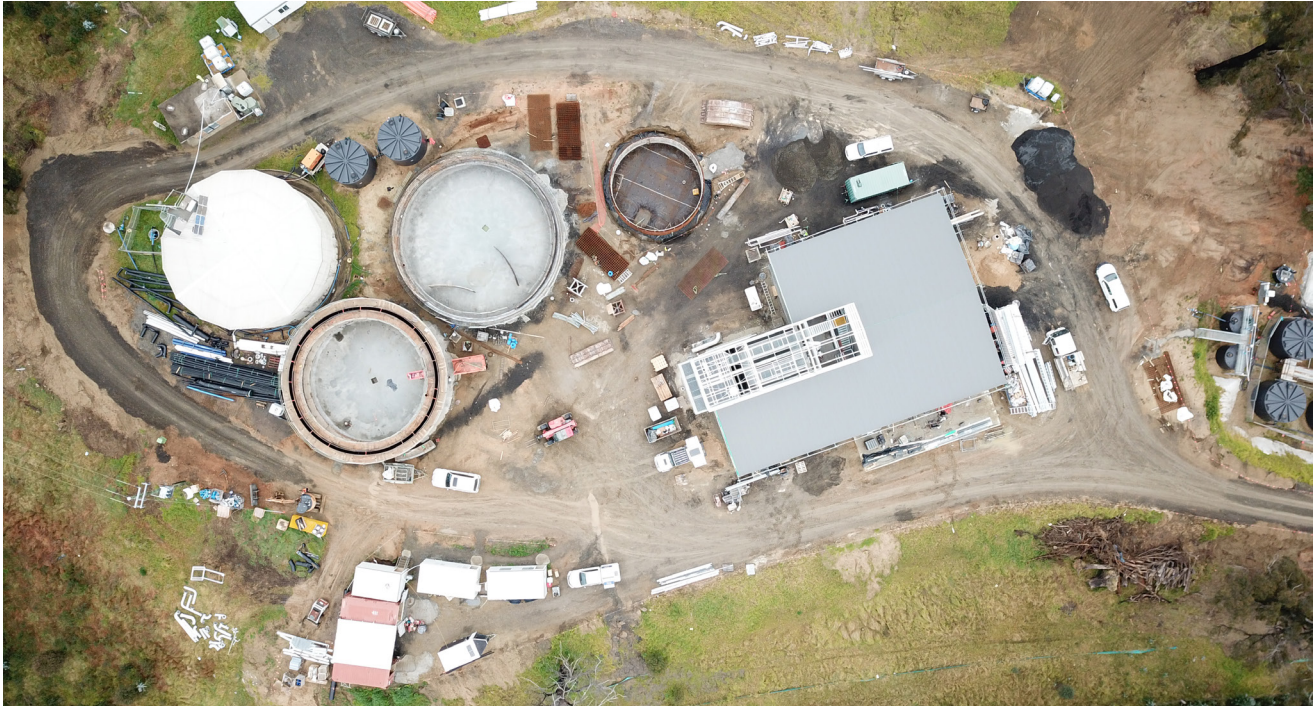
Brogo Bermagui Water Treatment Plant, NSW
