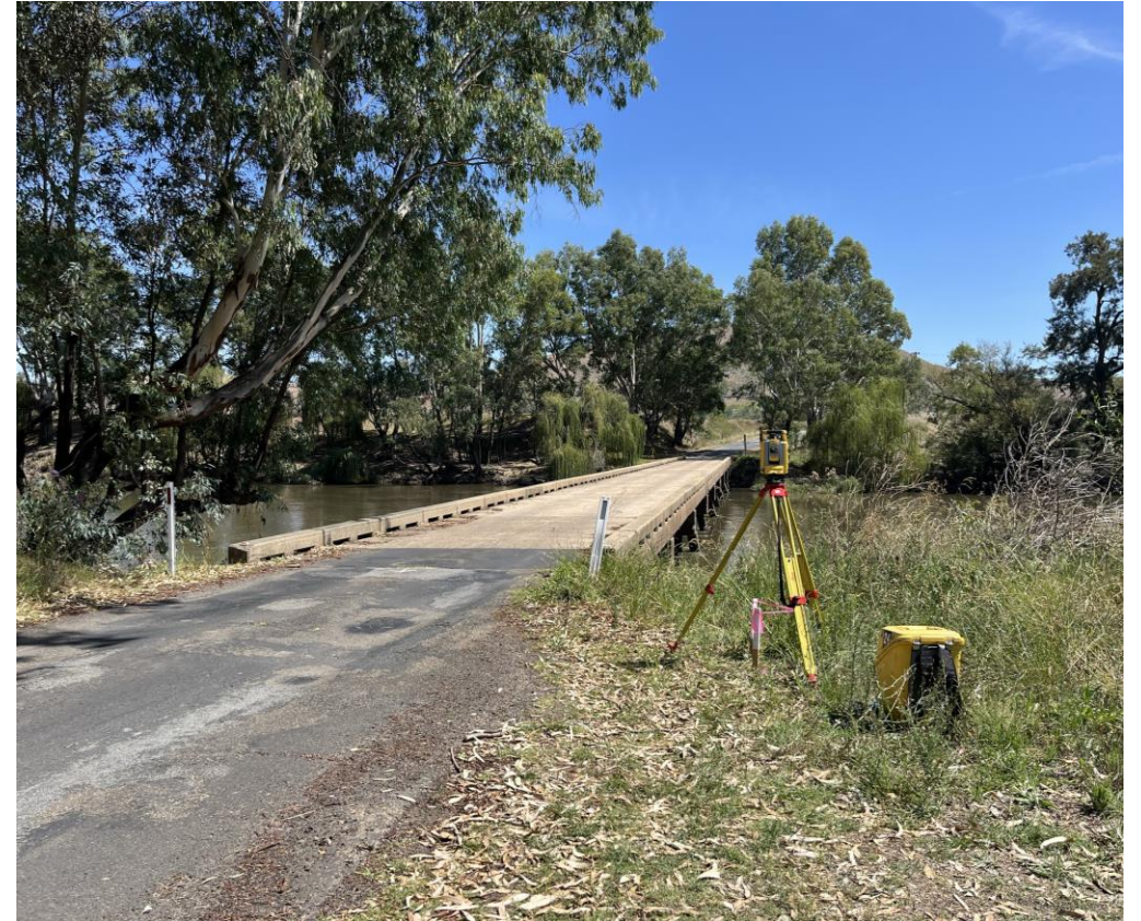
Survey work at Mundarlo Bridge, April 2025
