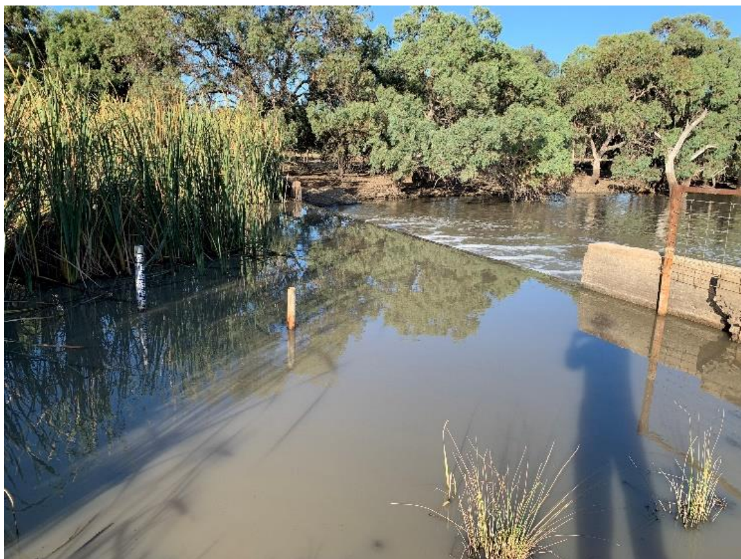
Figure 3.3 Existing condition of the project area, illustrating Forest Creek at Warriston Weir
