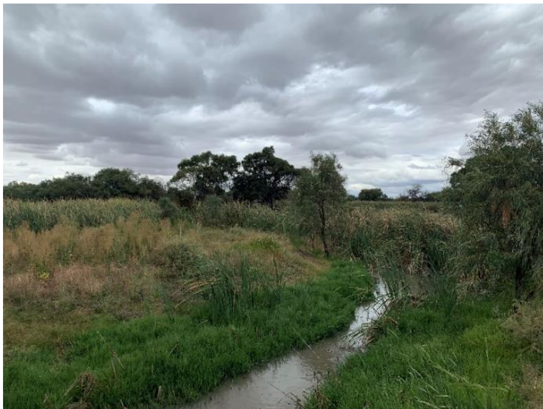
Figure 3.4 Piccaninny Creek downstream of culvert/road crossing
